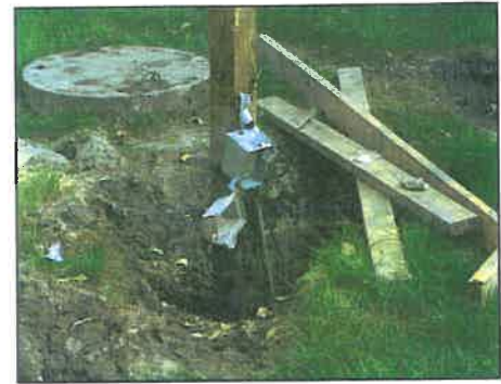
Flood damaged SSTS electrical box
