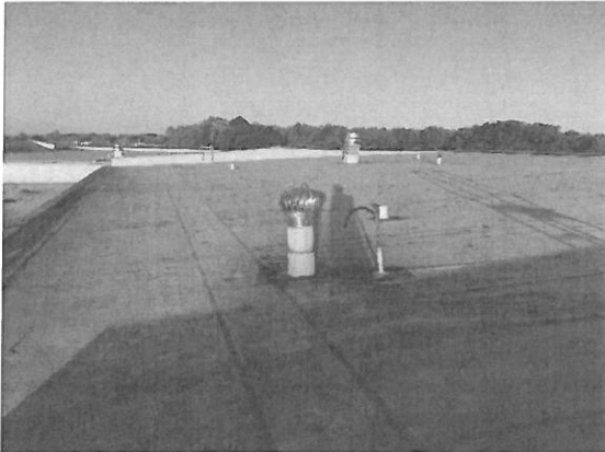
View looking west from the rooftop. Venting system wind turbine located in center of photo.
